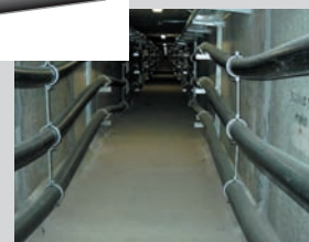
Opto-Power system installed on underground tunnel cable system. Circuit length 13 km. Single core cable length 40 km
